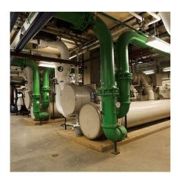
Satellite Utility Chiller Plant #3 Expansion, College Station Tx. Test, Adjust & Balance Project Size = Two new 3500 Ton Centrifugal Chillers and Cooling Total
